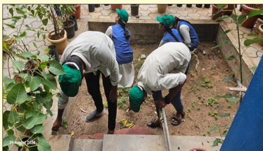
Waste removal from the soak pit
