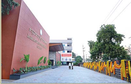
A panoramic view of Auditorium exterior
